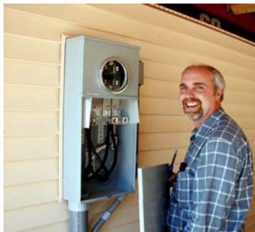
Next day building inspections
